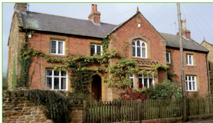
Estate cottages at Great Brington, built by E. Blore for the Spencer family in c.1848. Photograph B. McDonagh
