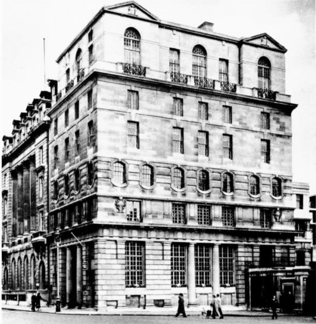
Figure 7: No. 68 Pall Mall (1928-9). Note the playful way in which the pilasters on the first floor appear to vanish into the rustication. Digital Image, available from: http://www.british-history.ac.uk/survey-london/vols29-30/pt1/plate-273 [assessed 15/04/16]
