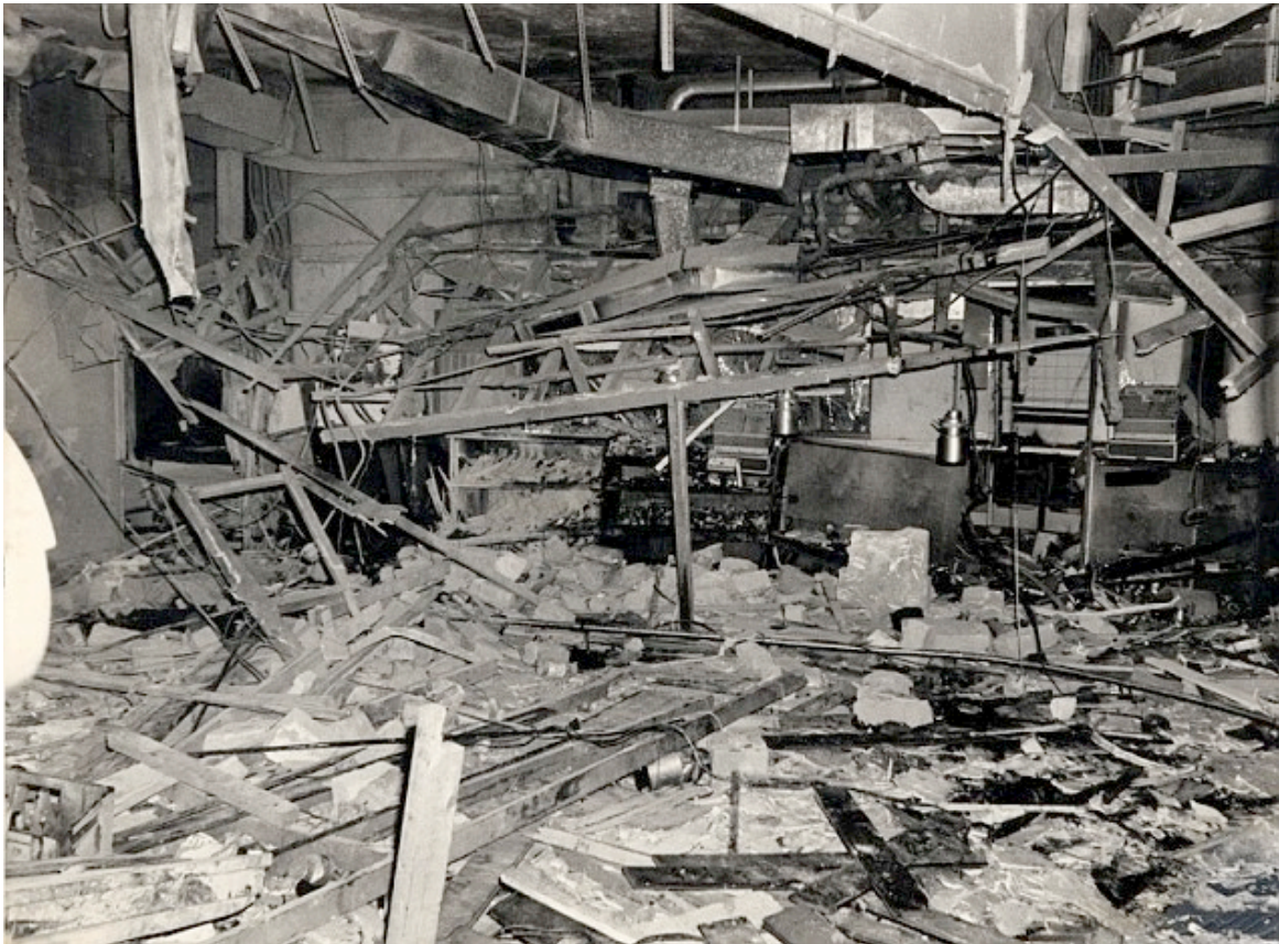
Figure 1. Damage to the Mulberry Bush pub 1
