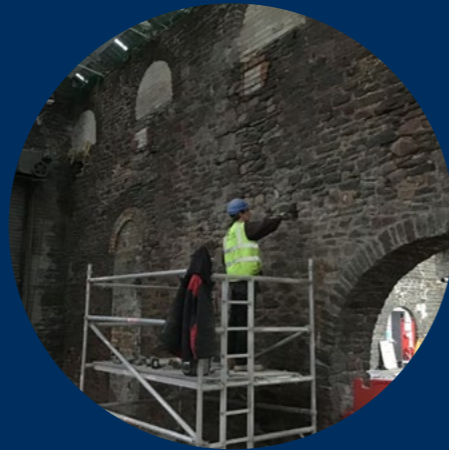
200 year-old walls exposed and repointed
