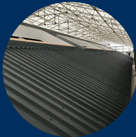
Original trusses secured and new roof revealed
