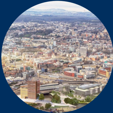
Planning permission secured October 2021
