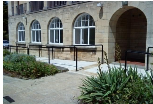
Ramp and front door
