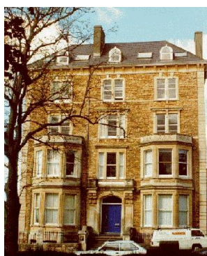
Canynges Hall, old facade – the front door some of you may remember
