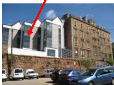
Canynges Hall - new extension
