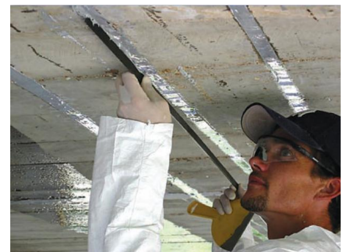
http://www.hughesbros.com Slab Retrofitting
